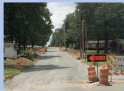
Country Club Road Major Street Rebuild
