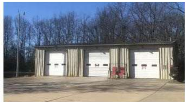
Sherwood Fire Station #3 at 10205 hwy. 107
