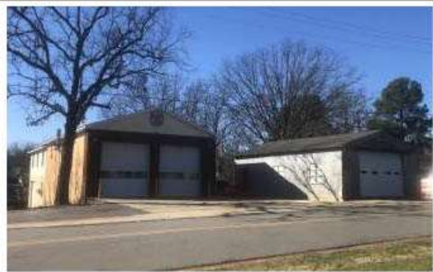
Sherwood Fire Station #2 at 505 Sherwood Avenue
