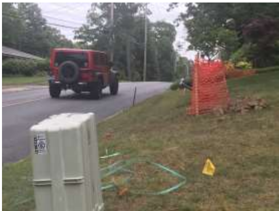
Utility Relocation work has started on Country Club
