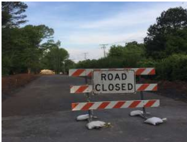
Kohl's Road: Still Less Than 500 Feet From Finished
